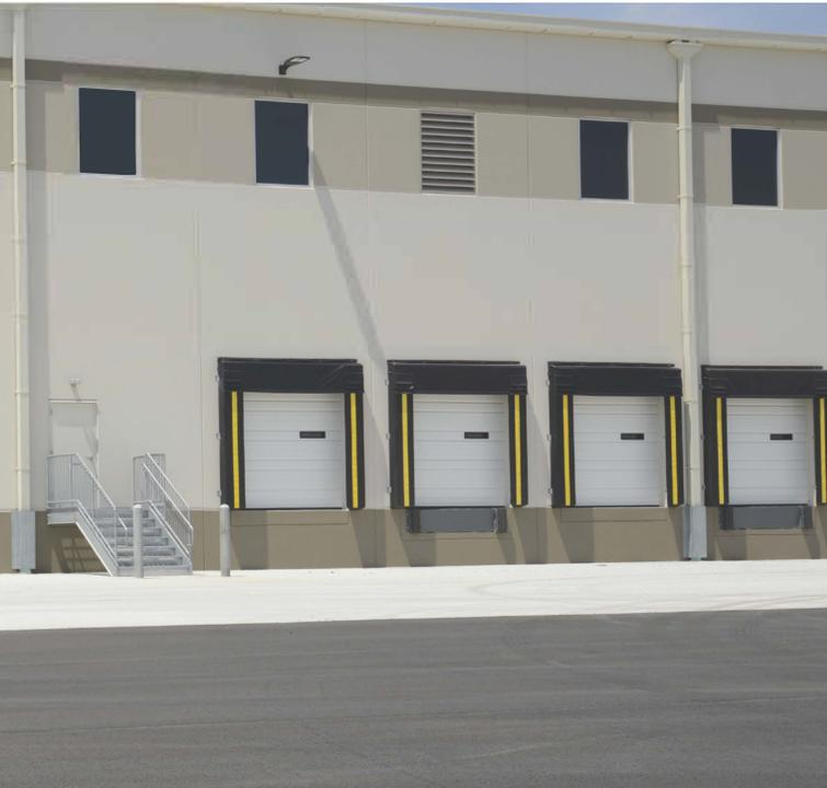
ProDoor's steel sandwich construction creates a strong and durable section that provides an insulated barrier from the harshest environments.
